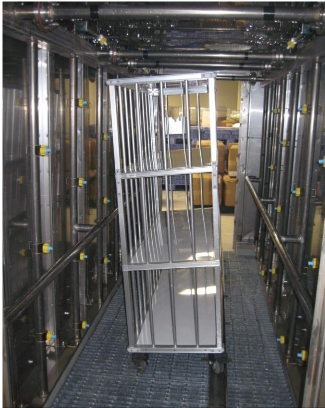
Raised cart guide helps drain cart and shelves
